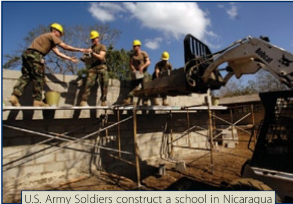
U.S. Army Soldiers construct a school in Nicaragua during a New Horizons exercise
