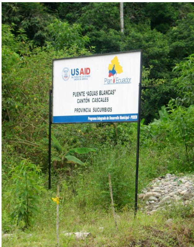
USAID AND PLAN ECUADOR BRIDGE PROJECT IN A BORDER COMMUNITY
